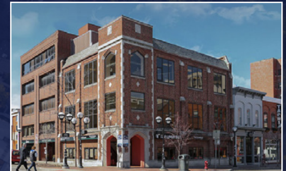
Federal Center Building 206 S. 5th Ave. 632 - 2,101 SF Available $28.00 PSF (MG)
